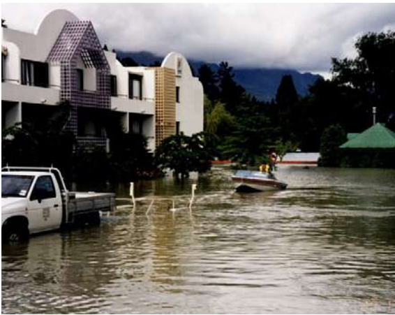
Above: Queenstown during the November 1999 flood. Image from Otago Regional Council
