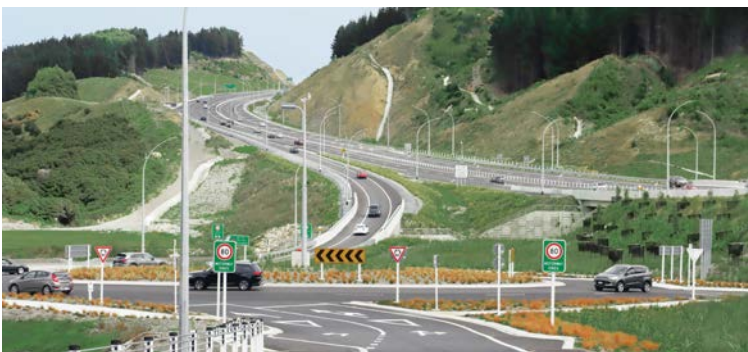
Transmission Gully Motorway Project
