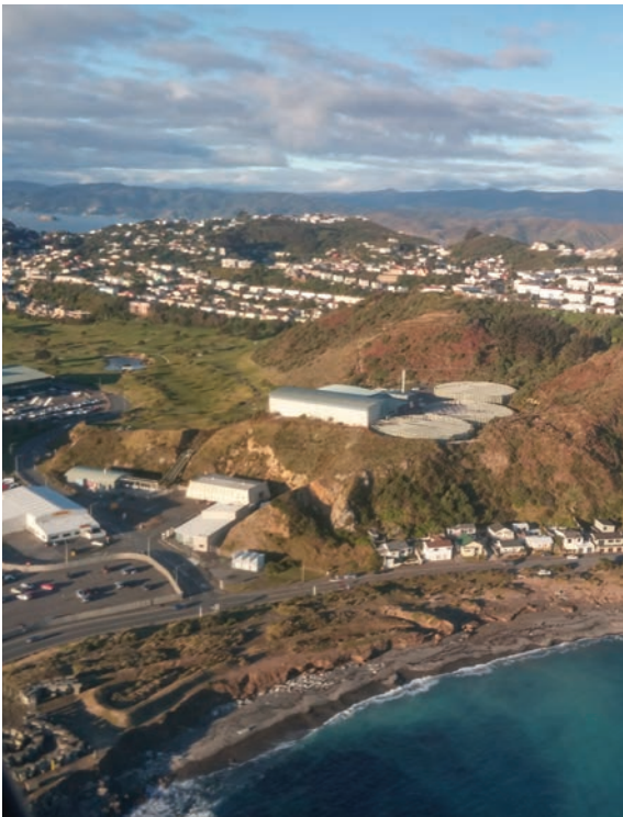
Moa Point Sludge Minimisation Facility
