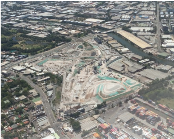
St Peters Interchange under construction.
