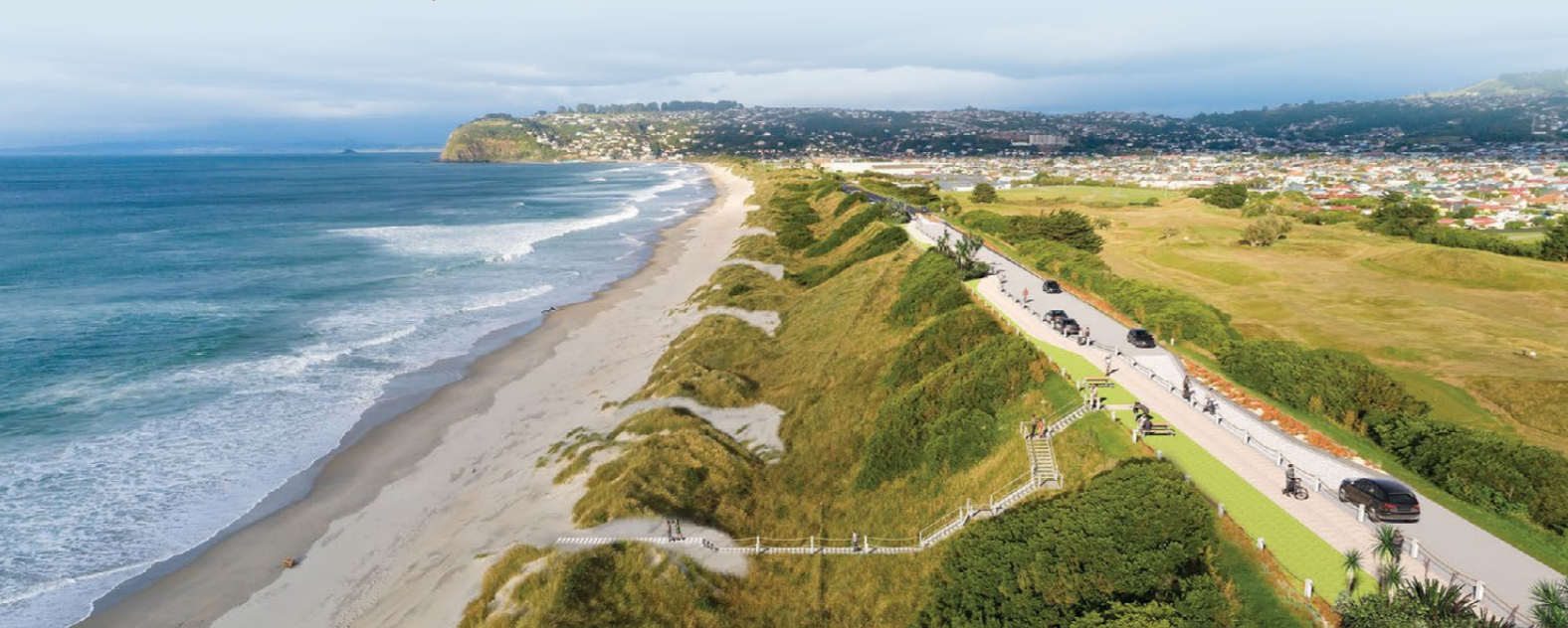
Concept visual of St Kilda improved access and dune management. Photo Credit: Dunedin City Council 2022.
